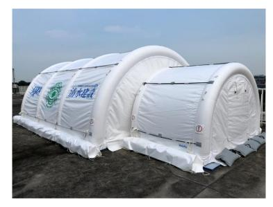
A possible solution to lunar habitation is an inflatable structure. JAXA, Tokyo University of Science, and Shimizu Corporation have investigated the possibility of inflatable structures on the moon for future lunar habitation. Through this demonstration module, we plan to test various aspects of human habitation.
