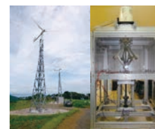
Monitoring of output power from multiple small wind turbines, and a prototype of a flywheel energy storage system
